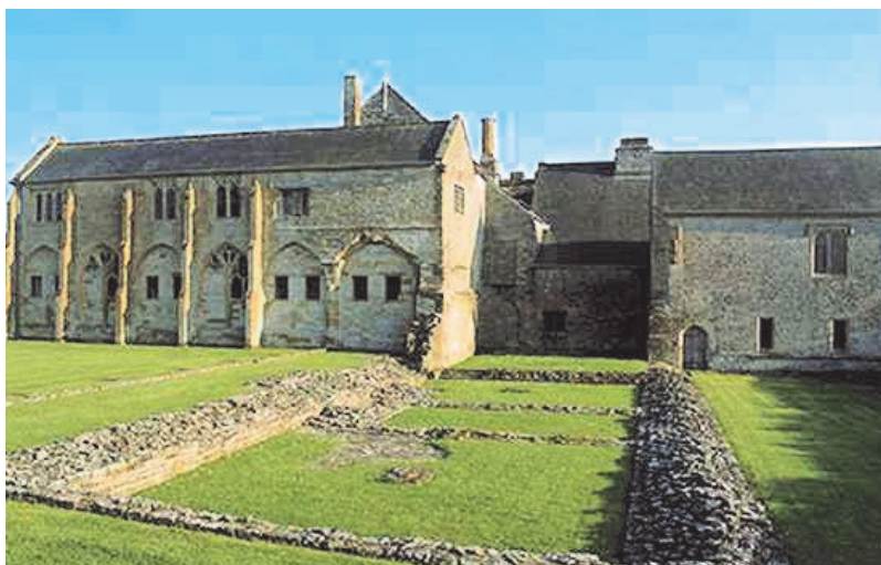
Muchelney Abbey in modern times. Remaining buildings stand behind the foundations of the abbey buildings levelled in 1538.
